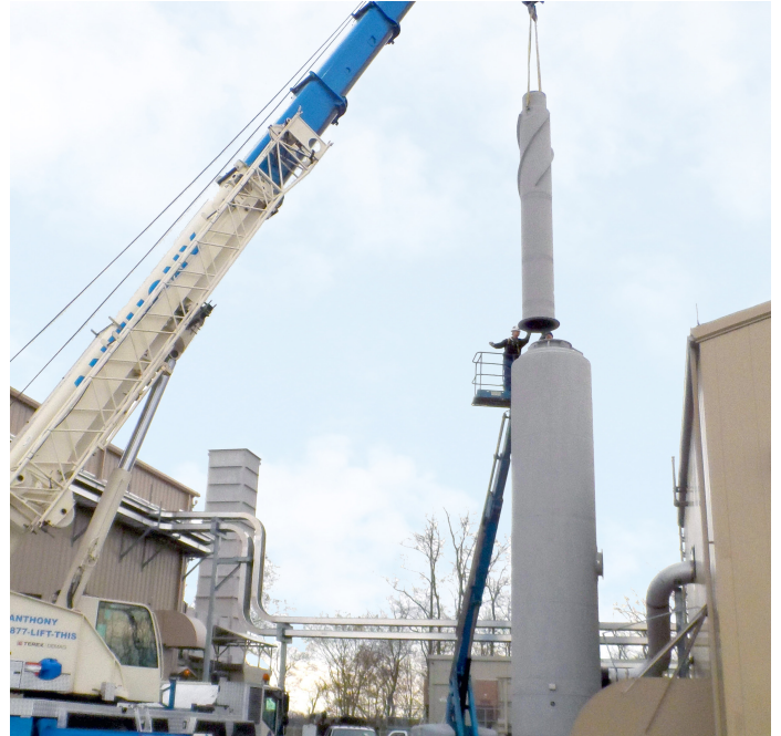
Exhaust stack installation
