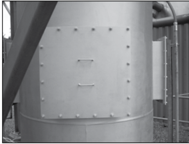
Figure 2: Proper positioning of catalyst access doors at the site is important for easy service.
