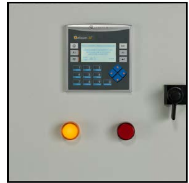
The GreenShield Catalyst Monitor provides data logging, text readouts and color-coded visual alarms.
