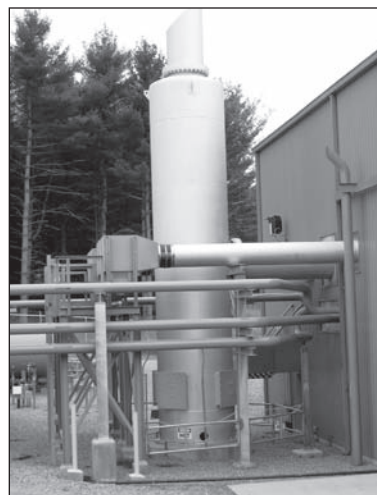
Figure 1: Universal provides a combination catalyst/silencer system that causes less engine backpressure.
